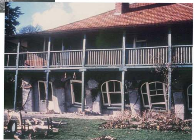
Damage to housing in the Cobb Road area in 1962 due to landslip. Image copyright WDDC.
