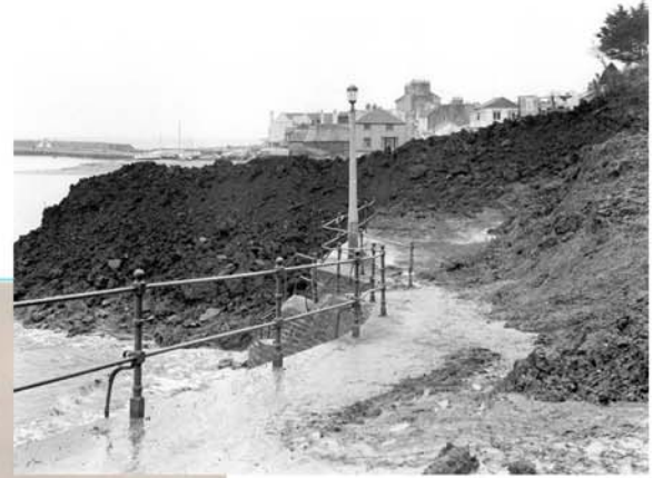
A landslide across Marine Parade in the 1960s, exacerbated by development work in the area. Image copyright WDDC.
