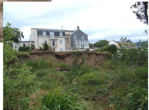
Damage to the garden of Stile House in Stile Lane due to a landslide in January 1999. Image copyright WDDC.
