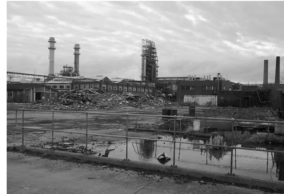
Castleford, West Yorkshire (Photo: Engineering at Cambridge)
