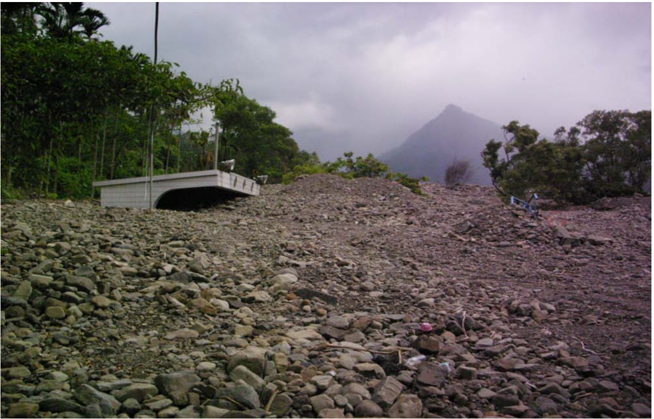
Fig. 22. Damage to Sanmin Elementary School from a Typhoon Morakot induced debris flow.
