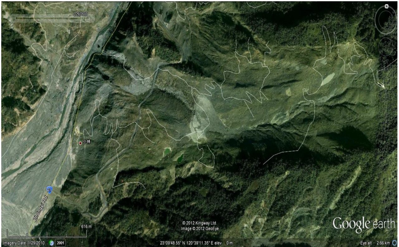
Fig. 31. Google Earth Image of the Site of the Xiaolin landslide 2009
