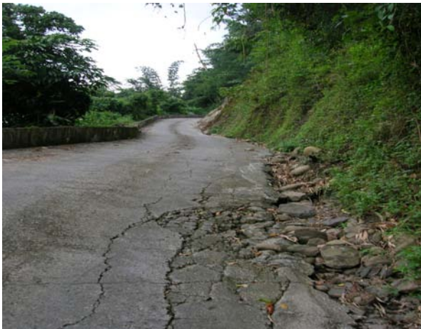
Fig.. 49 and 50 The road to the evacuation centre has fallen into disrepair (left) and crosses a landslide site (right).
