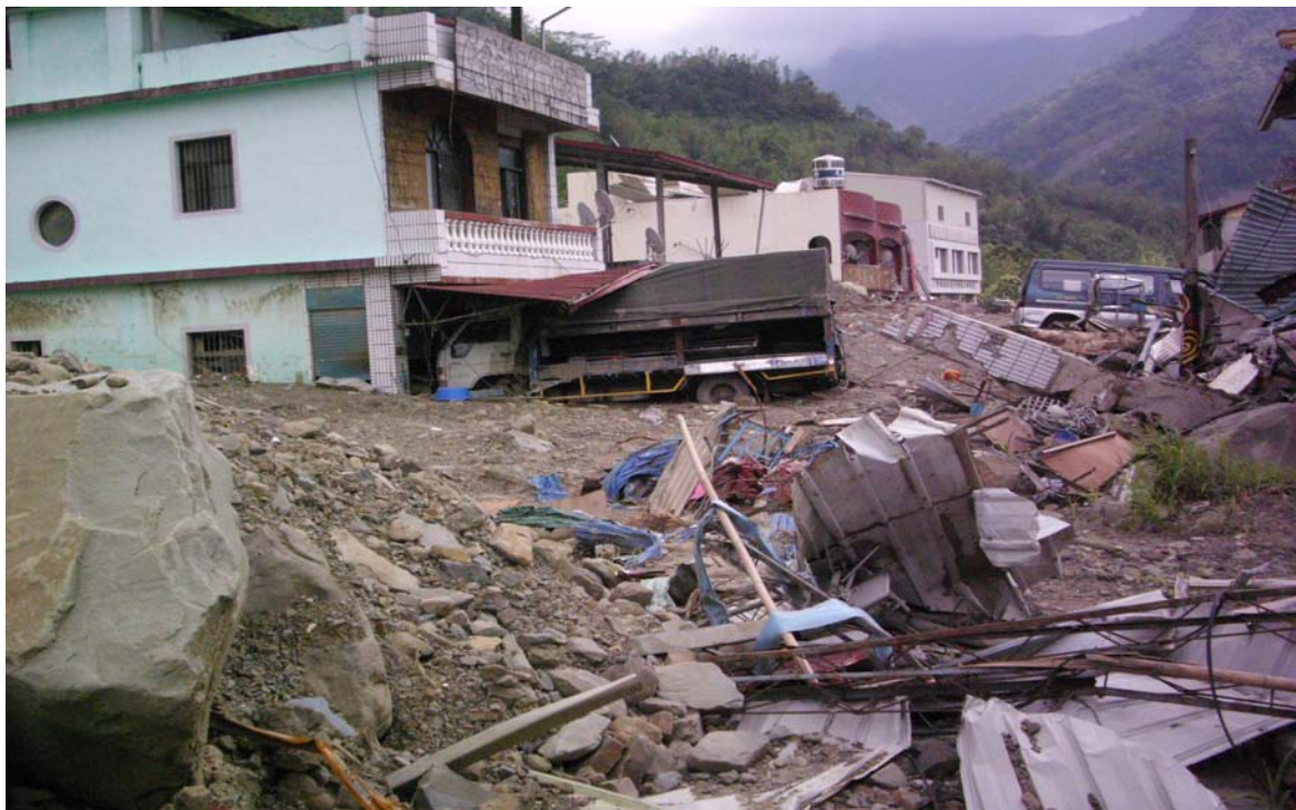
Fig. 23. Damage to Nangisalu Village from a Typhoon Morakot induced debris flow.
