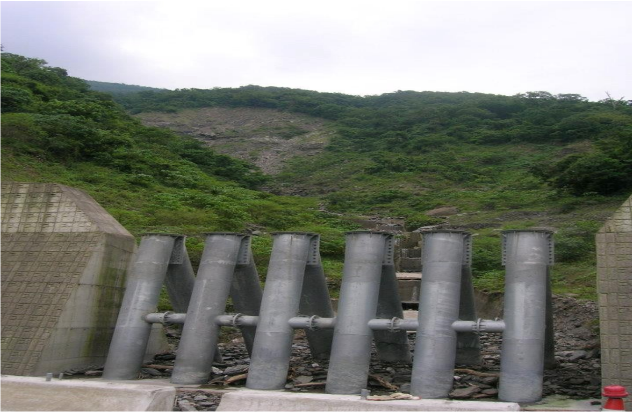
Fig. 12. Debris-flow protective barriers near Wanshan, Maolin
