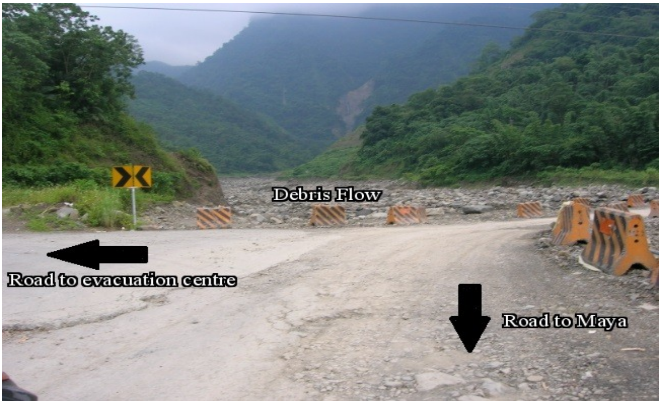
Fig. 51 The entrance of the road to the evacuation centre could be blocked if this debris flow is reactivated.
