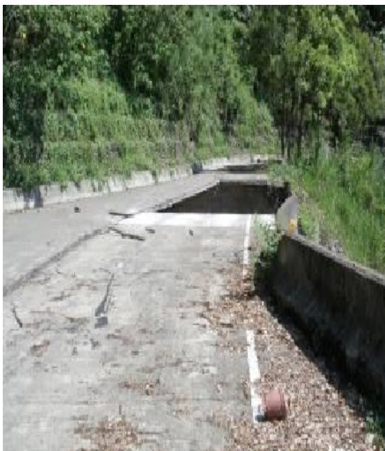
Fig. 28 and 29. Destruction of Highway 21 from Dakanua landslide.
