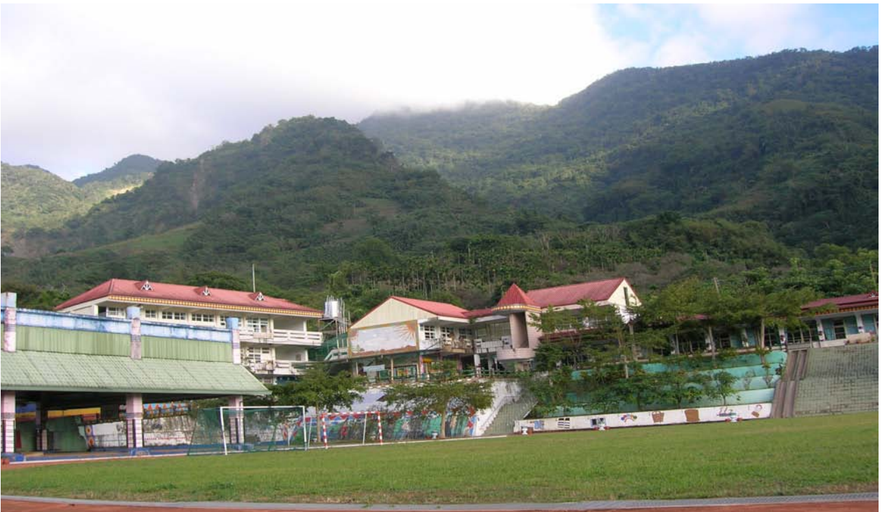
Fig.53. Dakanua Elementary school acts as the local evacuation centre.
