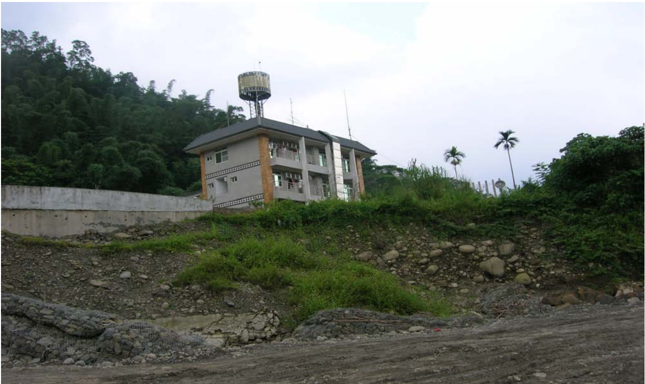
Fig. 55. Maya village Emergency Response Centre on the rapidly eroding banks of the Chisan River
