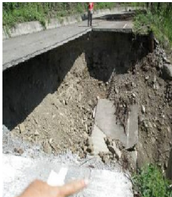
Fig. 28 and 29. Destruction of Highway 21 from Dakanua landslide.
