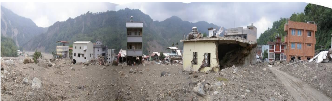
Fig. 21. Damage from a Typhoon Morakot induced debris-flow. Nangisalu village. 2009
