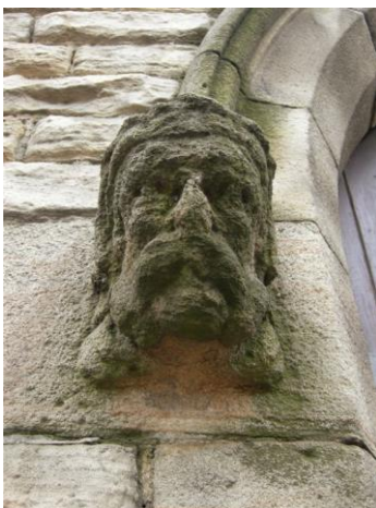
Figure 6 Acid rain damaged statue The definition of this statue has been lost as mildly acidic rain has worn down the features. (Source: Flickr Creative Commons User mafleen)
